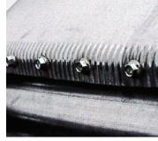
Rolled and crimped connections on the eaves and the hopper-to-sidewall matches corrugation of sidewall for extra strength and protection of contents.
